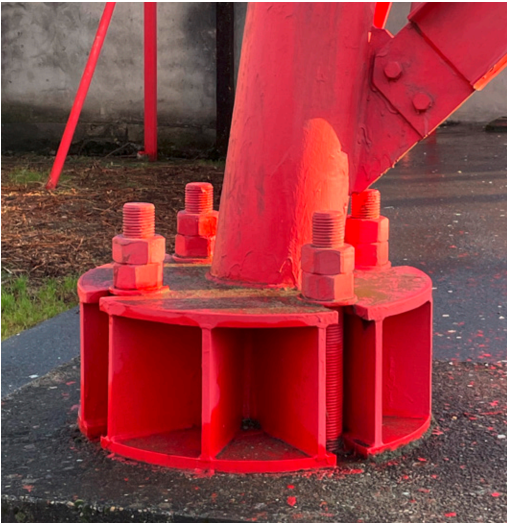
A ductile fastener requires adequate elongation length and elongation at break.
